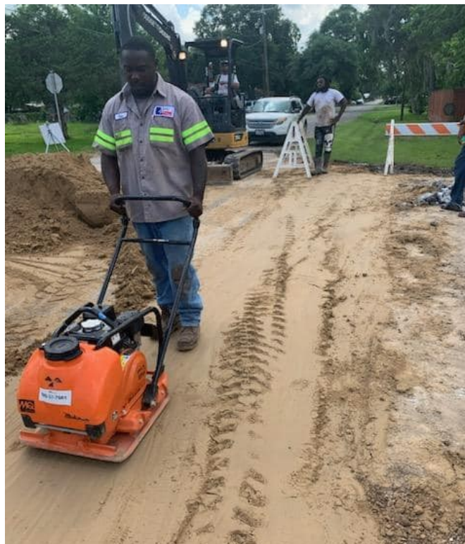
Crew Leader training Public Works staff on road repair.
